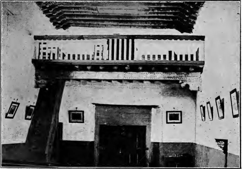
INTERIOR OF THE CHURCH OF SAN MIGUEL, SANTA FÉ Showing the gallery and carved Vigas , or round timbers of equal size
